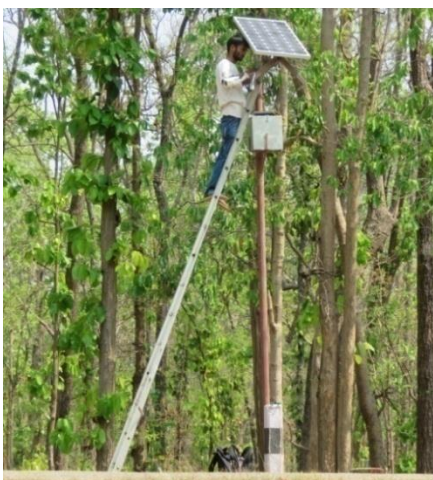
Photo 11: Solar panel installation for fence.
